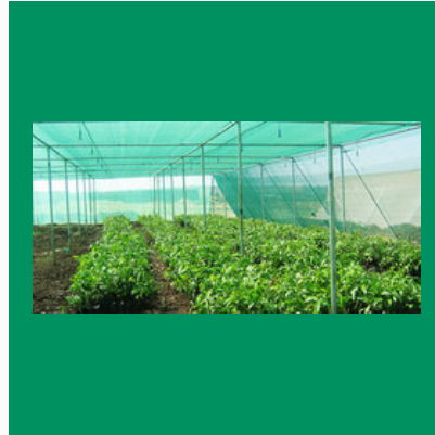
Flat Net House Structure
