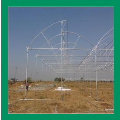
Polyhouse Construction Services
