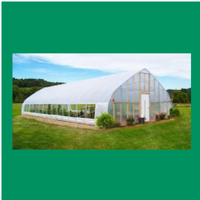
Film Greenhouse Structure
