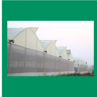
Poly house Structure
